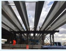
I-25 bridge girders are precast concrete beams and vary from 72 to 155 feet in length and are an integral part of the bridge deck support structure that carries the traffic. A 500-ton and a 300-ton capacity crane were used
